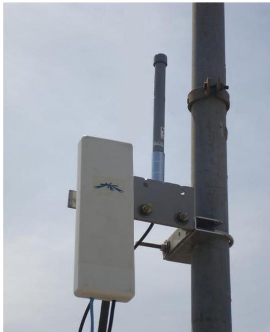
Figura 2. Nanostation e Antena 8dB
